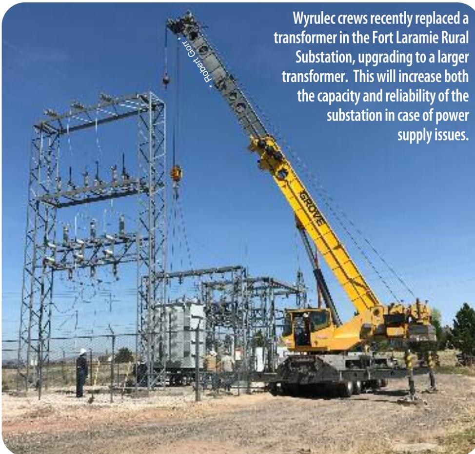
Wyrulec crews recently replaced a transformer in the Fort Laramie Rural Substation, upgrading to a larger transformer. This will increase both the capacity and reliability of the substation in case of power supply issues.
